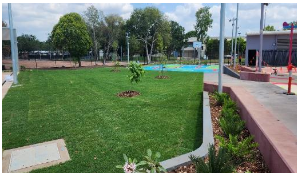
Laying of turf for the entertainment area.
