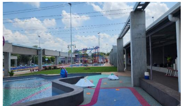
Completion of the water play area with turfed connection areas
